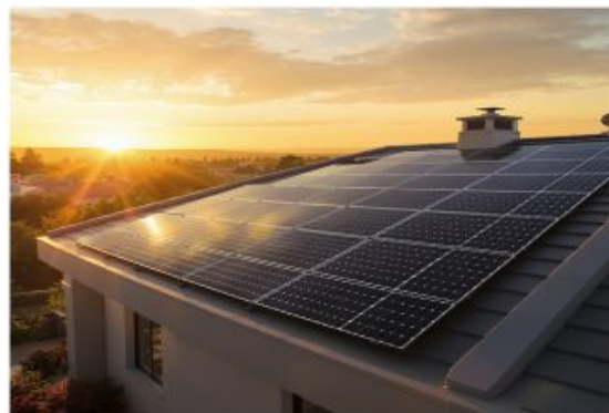
Solar Panels / Solar Roof Renewable energy generation
